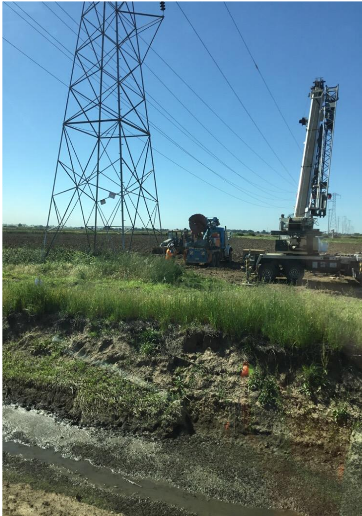
Photo 1: Tower crews preparing to drill and install a foundation at site 19/142.
