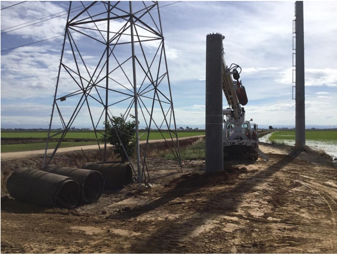
Photo 2: Crews installed a new pole base at site 27/199.
